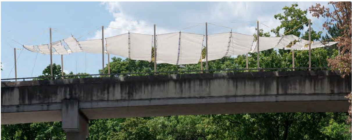
Figure 35 - Shading demonstrator on St. Jakobus bridge in Neuperlach.
